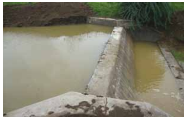
Check Dam built in the Medak Project
