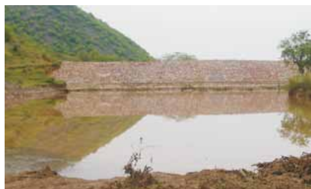
Water recharge structure at Neemrana Rajasthan
